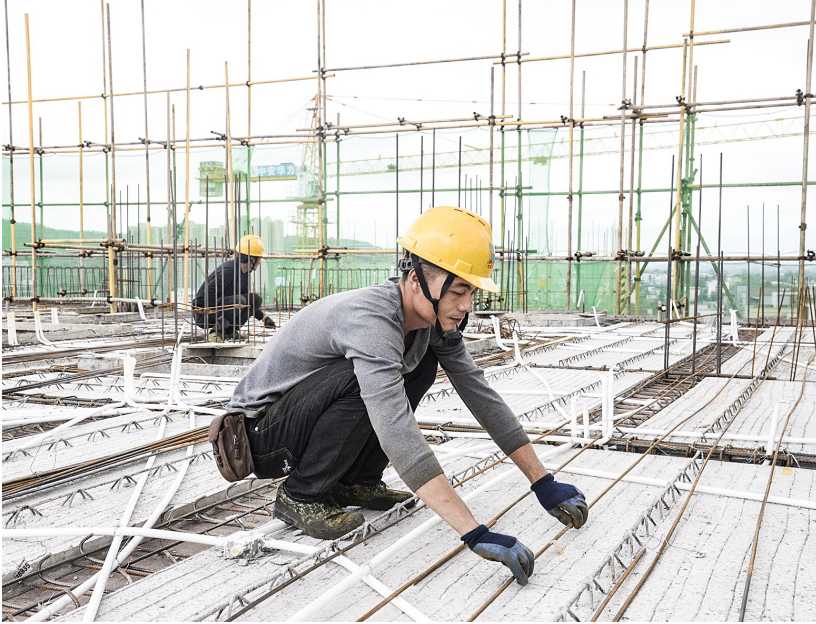
工人绑扎钢筋
